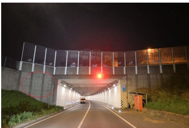
CuGa0 Left wing wall Axis 0 1216 other cracks Entire wall. Surface microcracks.
